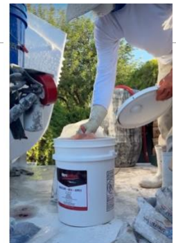
Mixing Operator Measuring SetNCure & Adding to Mixer
